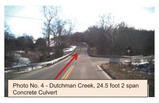
Dutchman Creek is not structurally deficient or functionally obsolete. The bridges at Plum Creek and Elk Creek are not structurally deficient, however, they are functionally obsolete. A bridge structure with a Sufficiency Rating below 50.0 is considered for possible replacement by the Transportation Cabinet using federal bridge funds. Based on this, none of the bridges are eligible for replacement at this time.
